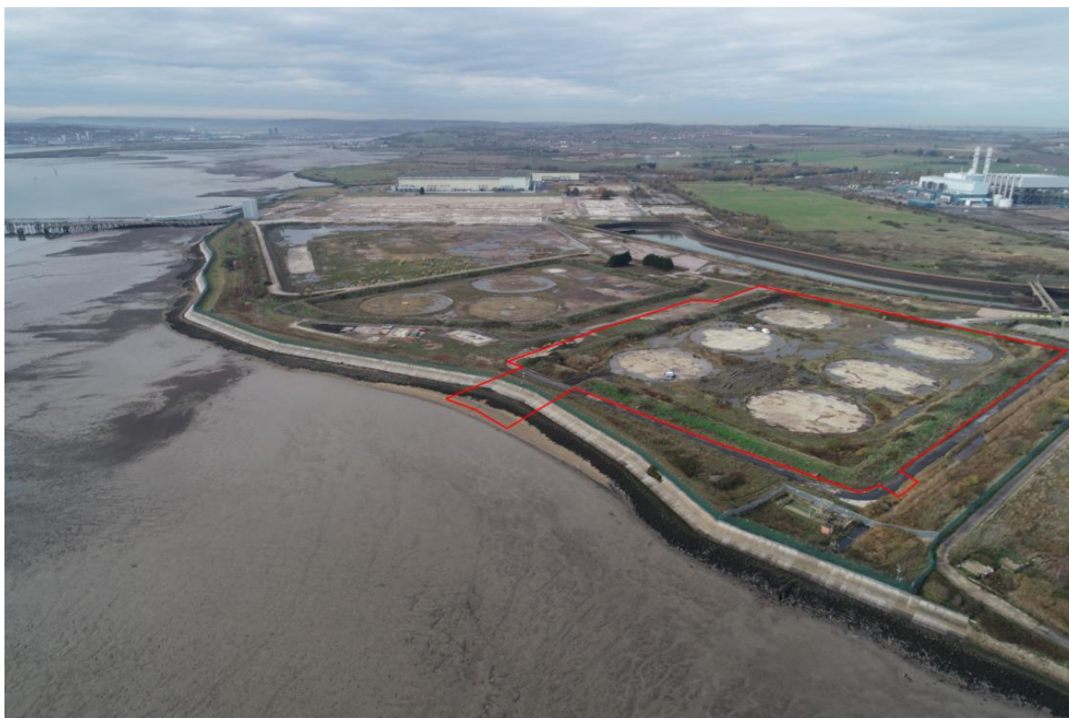
Photograph 2-3 The demolished Kingsnorth Power Station and surrounding areas, with flood defence seawall and mudflats of the River Medway (west facing)
